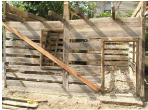
springhouse dismantled by Denlinger Fisher Builders of Paradise
